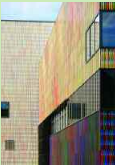
MUSEUM BRANDHORST - MUNICH, EXTERIOR
